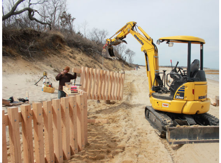
PANELS ARE ASSEMBLED AND LAID OUT
