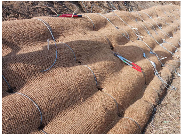
ARRAY IS BLANKETED AND ANCHORED IN PLACE
