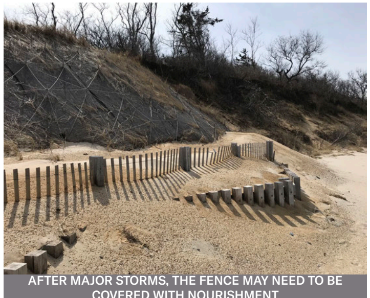
PANELS ARE ARRANGED IN A ZIG-ZAG FORMATION TO HELP CAPTURE WIND-BLOWN SEDIMENT
