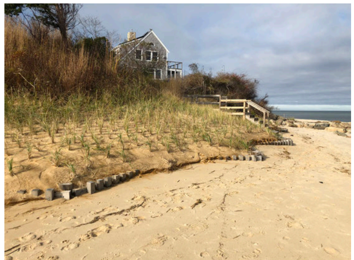
ROLLS CAN BE PLANTED INTO TO GET VEGETATION & ROOT SYSTEMS ESTABLISHED
