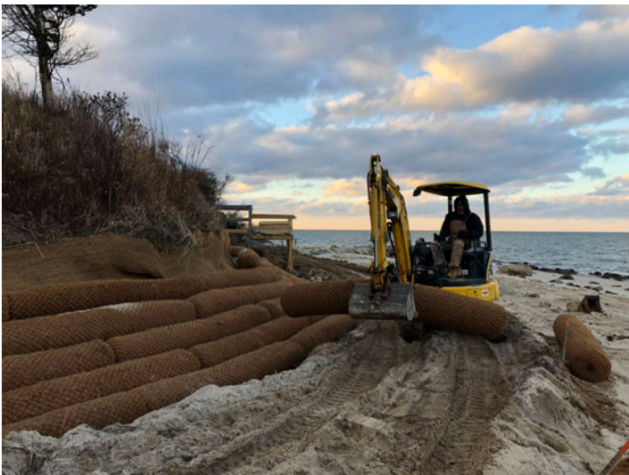
ROLLS ARE STACKED VERTICALLY ALONG THE FACE OF THE BANK TO RESTORE A DESIRABLE SLOPE
