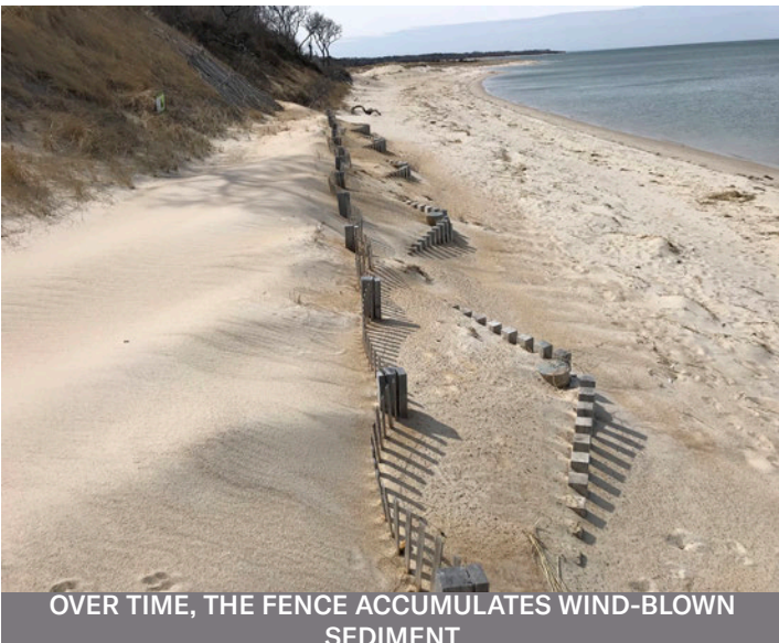
PANELS ARE ARRANGED IN A ZIG-ZAG FORMATION TO HELP CAPTURE WIND-BLOWN SEDIMENT
