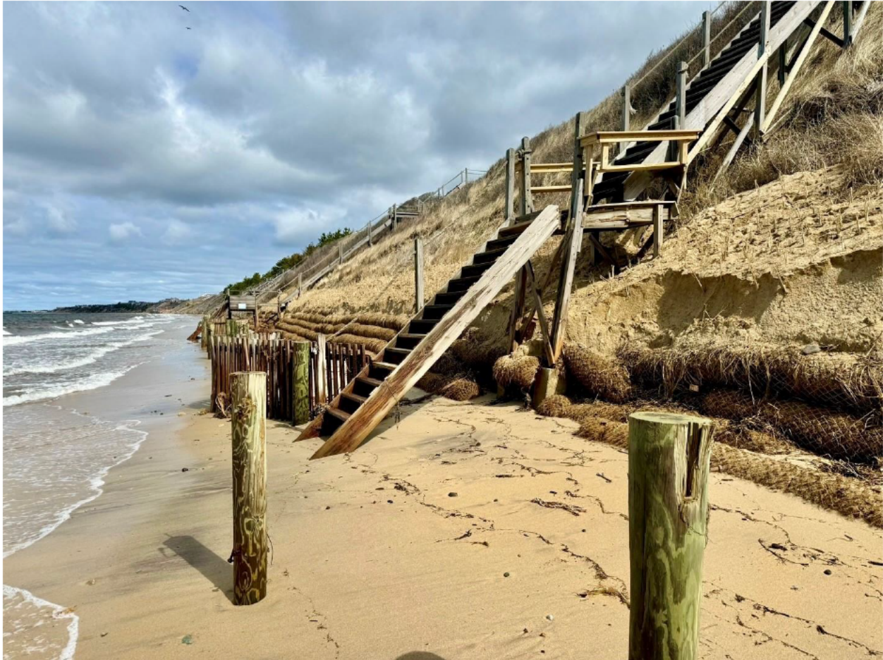
Condition of array next to stairs, there is significant slumping.
