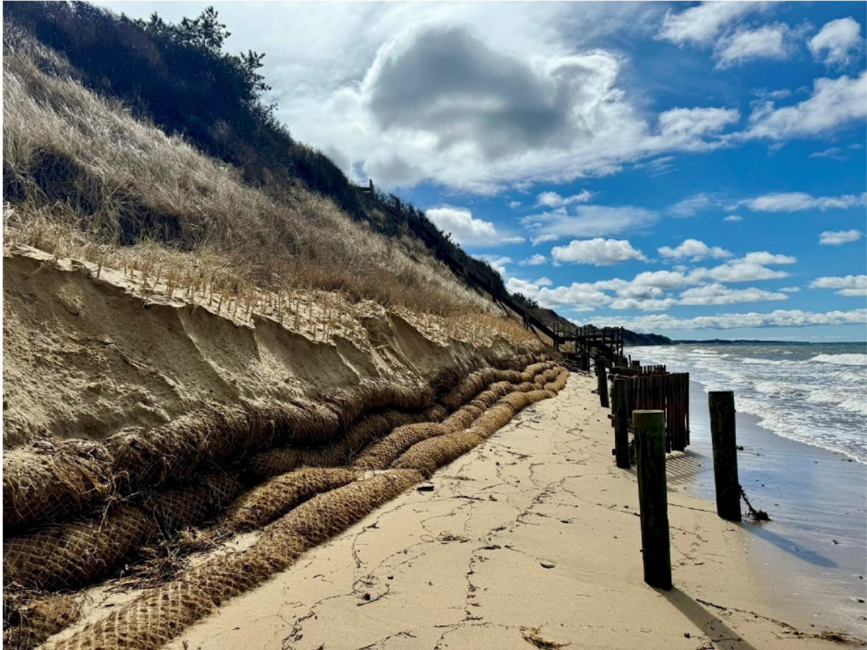
Condition of array showing all 4 rolls exposed and slumping of installation from overtopping of array and lack of a stable toe.
