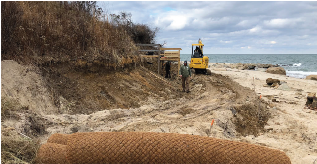
COASTAL BANK PREPPED & TRENCH DUG FOR FIRST FIBER ROLL
