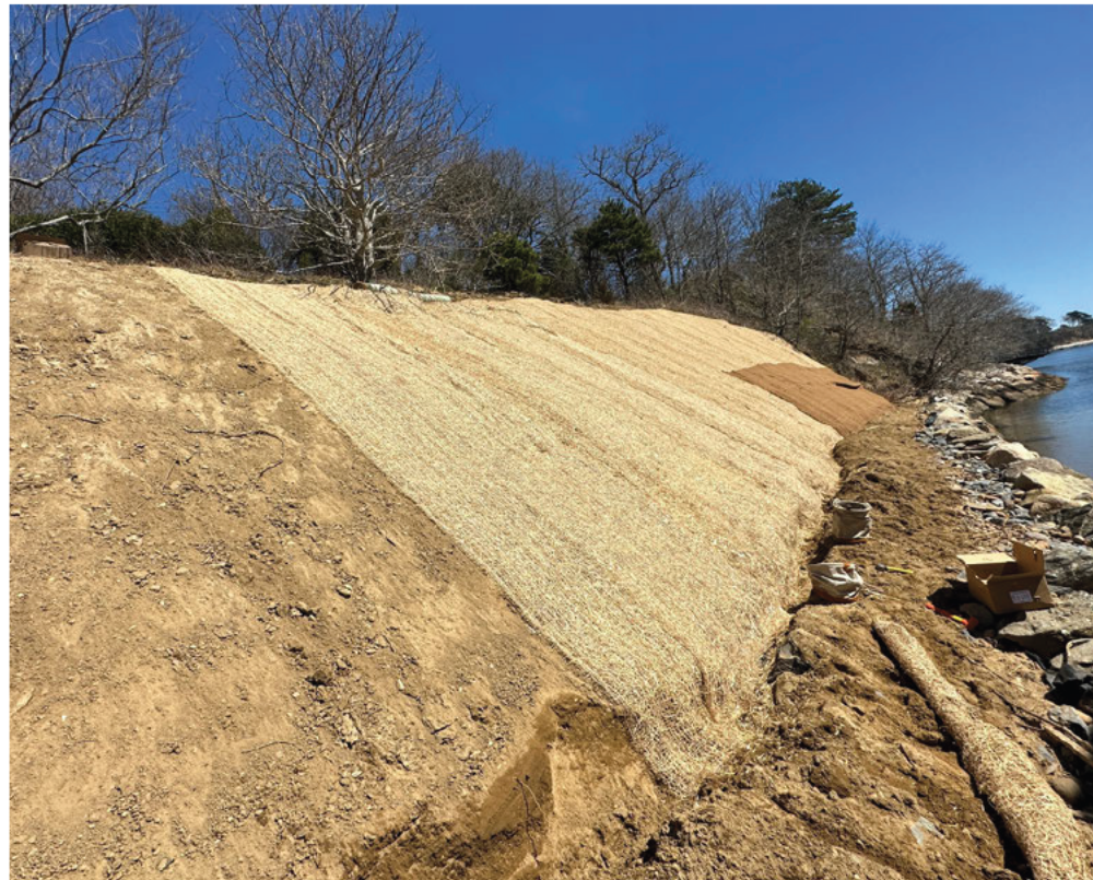
INITIAL BANK STABILIZATION AND BLANKETING WORK IN PROCESS
