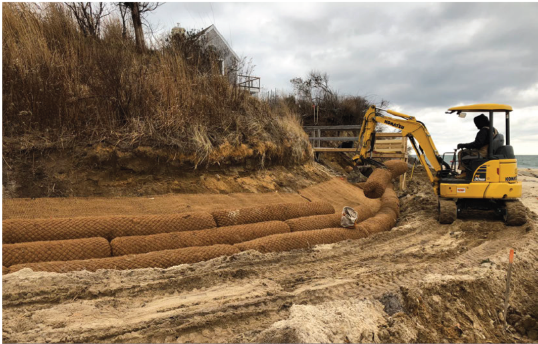
FIBER ROLLS BEING PLACED
