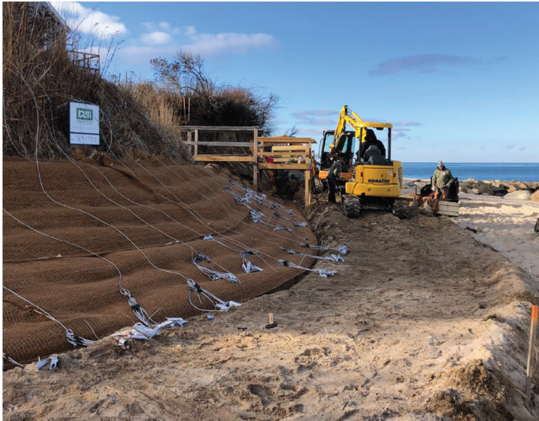
WHIPS & ANCHORS IN PLACE
