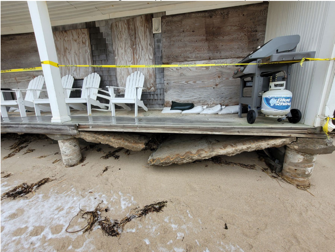
Photos 7 & 8: Winter storm damage; easterly portion of foundation exposed (1/16/24).
