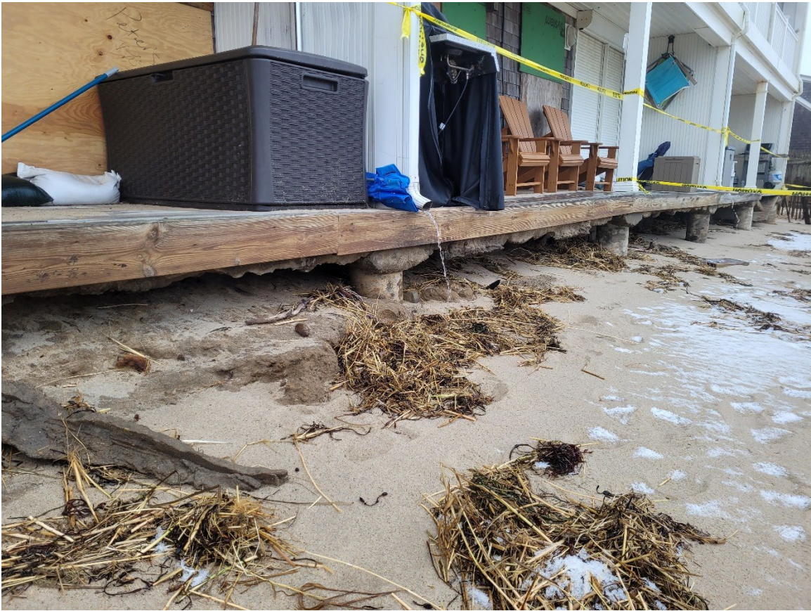
Photos 7 & 8: Winter storm damage; easterly portion of foundation exposed (1/16/24).
