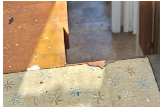
Sheet flooring and board flooring at second level, crumbling and failing from age.
