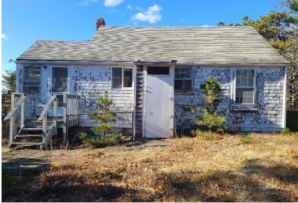
View showing wooden steps into kitchen addition that are rotting due to age, and an exterior accessed shower stall attached to the back of the building.
