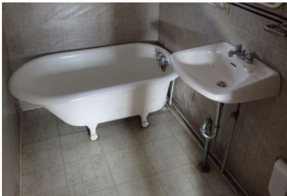
Sink and bathtub, both with non compliant hardware. Toilet is also present as well in this bathroom.
