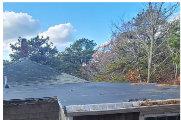
View of rear addition membrane roof in relation to original asphalt shingle roof. Evidence of ponding can be seen in the membrane roof, with vegetation build up in the gutter as well.
