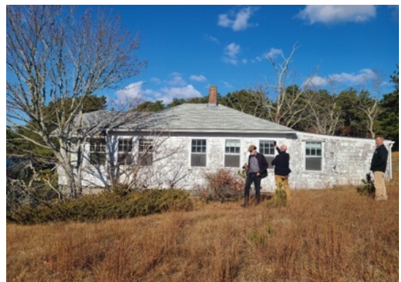
Southern face of cottage, front and rear additions are apparent. This face is missing at least 50% of its paint.
