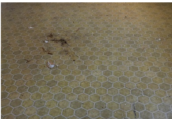
Worn and damaged sheet flooring.
