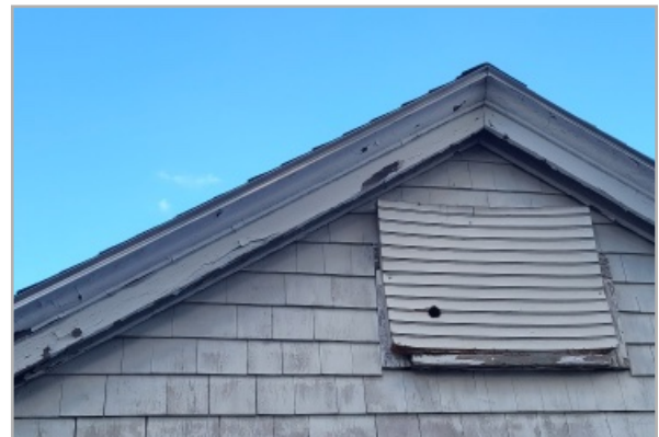
A view of the rake condition of the original roof. A louver is located at the peak, and has deflected out of its penetration. The rake shows sign of mold between the fascia board and siding.
