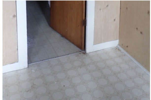
Sheet flooring with signs of degradation throughout and crumbling at the edges.
