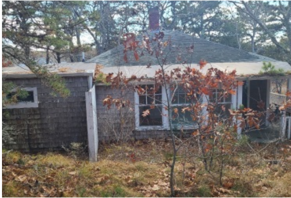
Northern face of the buildin. Most windows are single paned wood windows lacking aluminum storms. A few windows have wood framed storms.
