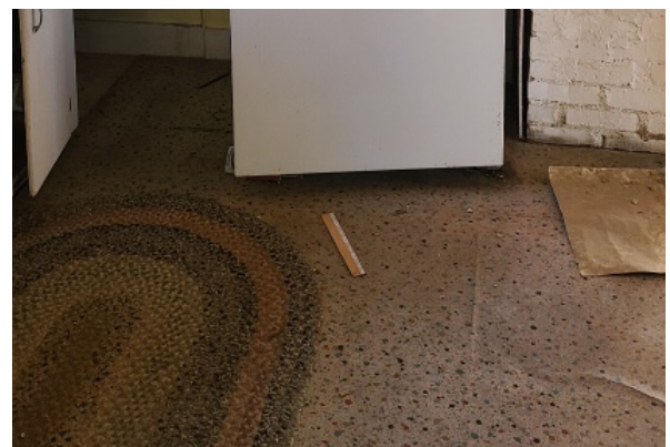
Sheet flooring that is badly worn with visibly evident floor deflection throughout.
