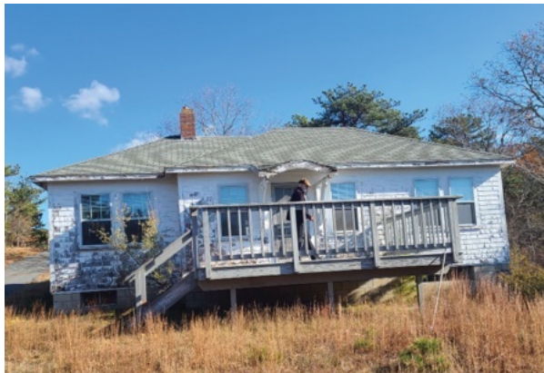
Front view of cottage, CMU foundation has two window penetrations just above grade. The paint is peeling throughout.
