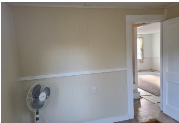
Painted plaster wall with trim at base, mid, top, and about doorways. Paint is yellowing due to age.
