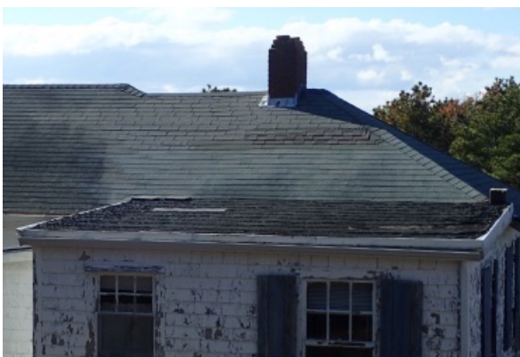
Poorly constructed addition with degraded asphalt singled low pitched shed roof.
