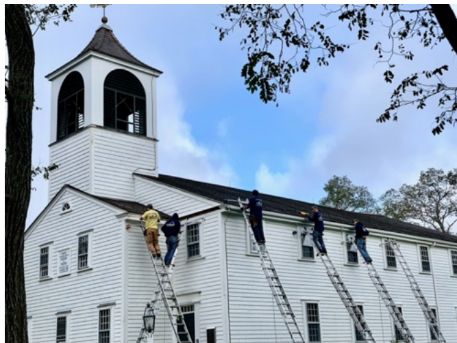
Replacing the gutters and repainting and painting the fascia boards, 2019.
