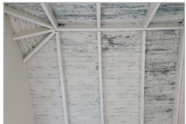
Interior of roof in front porch addition, with peeling paint and signs of water ingress.
