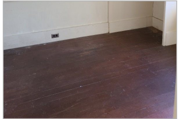
Wood flooring in bedroom is in fair condition. Non-grounded electrical outley located in baseboard.
