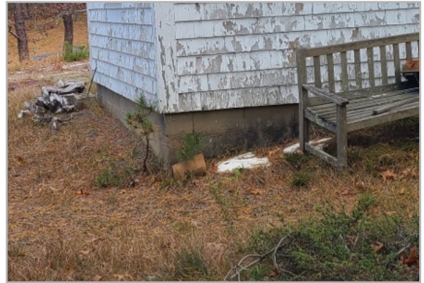
View of CMU foundation at South West corner, vegetation is beginning to encroach and the presence of a tree sapling suggests root penetration.
