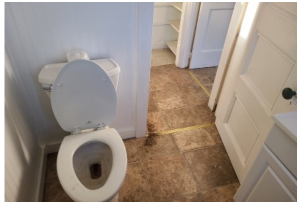
Toilet fixture and sink, the layout of this bathroom is non-compliant with accessibility codes.
