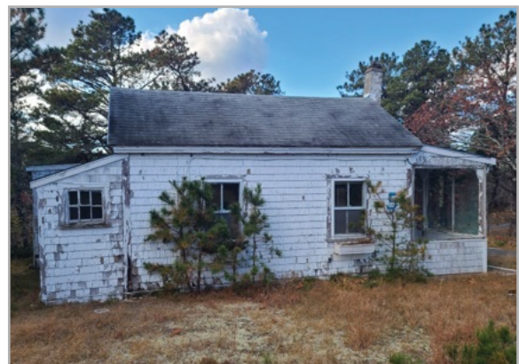
Building siding paint is peeling throughout with rotting deteriorated shingles and wood trim boards.
