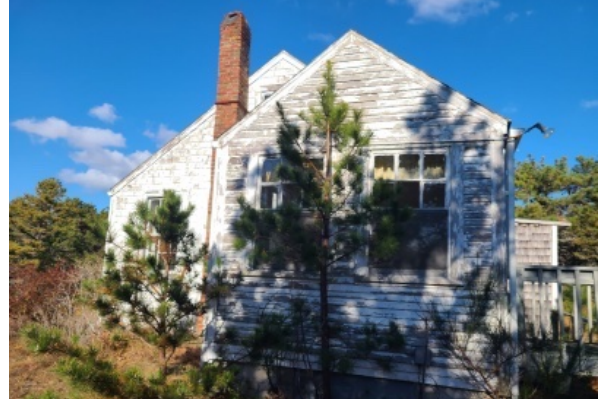
Southern face of the building kitchen addition with newer windows than the rest, but still insufficient due to age.
