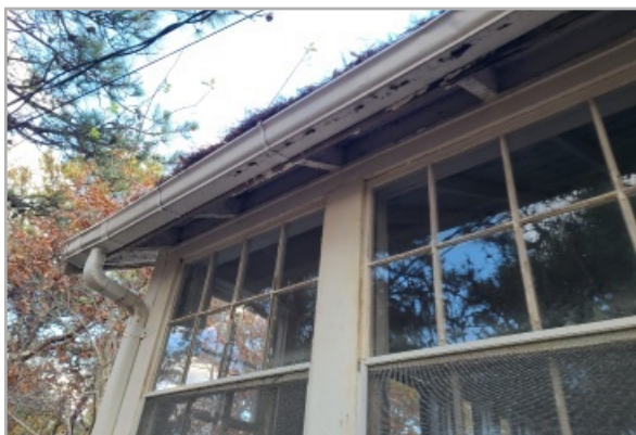
View of exposed and rotting eave with aluminum gutters sagging from the weight of accumulated organic matter supporting live vegetation.
