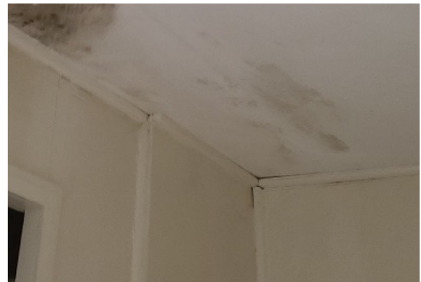
View from the interior of water damage and mold seen in the ceiling indicating multiple areas of water penetration into the roof.
