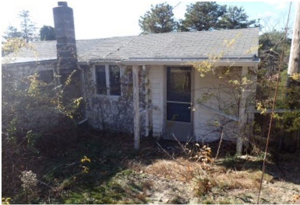
East elevation has excessive vegetation overgrowth that has penetrated the shingles in some areas.
