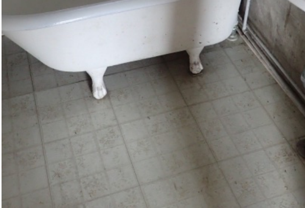
Sheet tiling in bathroom that is crumbling at the edges and seams.
