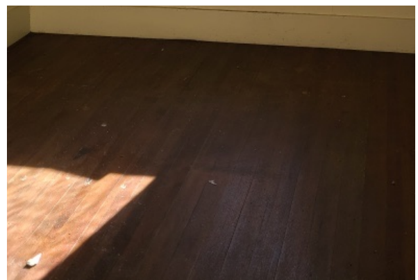
Hardwood flooring needs restoring, and has a slight pitch indicating foundation settlement.
