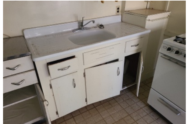
In counter sink and cabinet storage underneath. The cabinets and drawers could not close due to warping and the deflection of the floor structure below.
