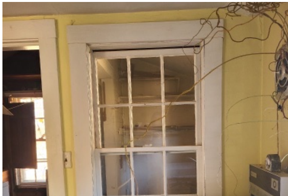
Exterior window that became interior with the side addition. To the right is a through-wall exhaust fan with vegetation penetration.
