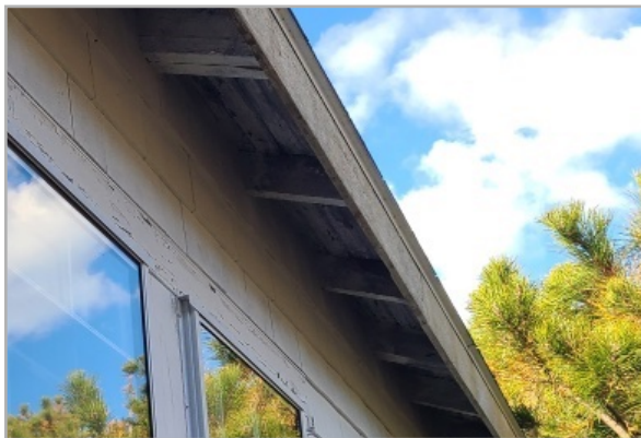
Exposed roof rafters at eave show signs of rot, and peeling paint on fascia board.
