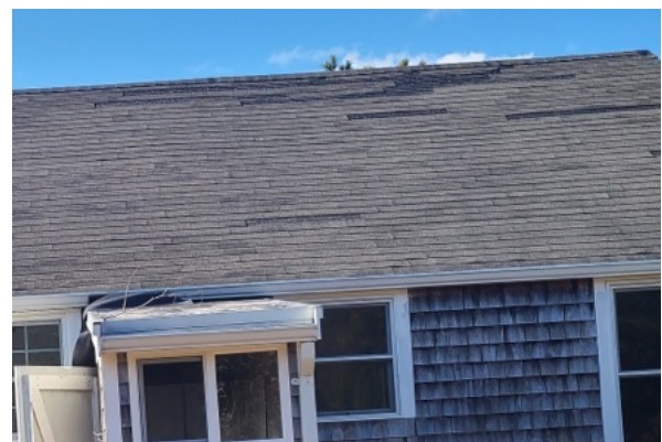
Asphalt roof generally is failing, and the shower stall addition has failed at the connection to the main structure.
