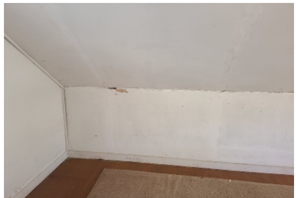
Variable wall heights at second level with trim board at borders, paint is chipping and peeling throughout.
