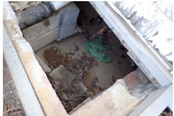
Access to foundation crawl space, the foundation of CMU and wood members can be seen.
