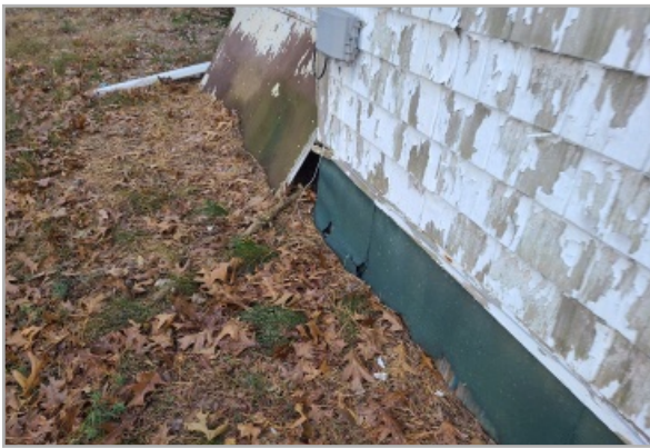
Deteriorated painted plywood foundation skirting.
