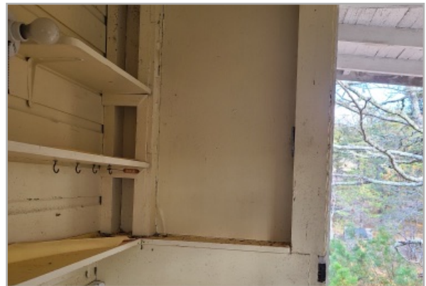
Kitchen addition wall has an unfinished interior with chipping and peeling paint. Due to the age of the structure, lead paint is assumed at all painted surfaces.
