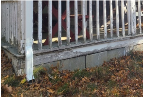
CMU on grade foundation for porch addition is an insufficient structure, and the wood framing is in contact with the ground on the northern side (left).
