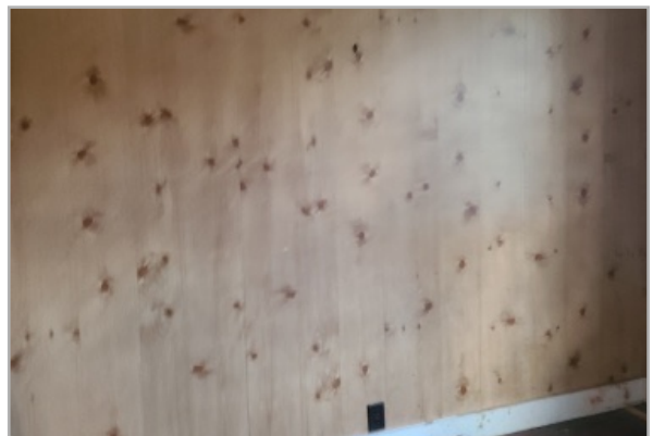
Wood panel walls, naturally stained with a contrasting base board. There are signs of mold and mildew growth in some areas.
