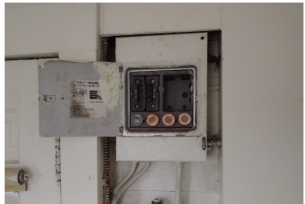
Conduit box with original fuses is non compliant and must be removed and replaced with up-to-date fixture and wiring.
