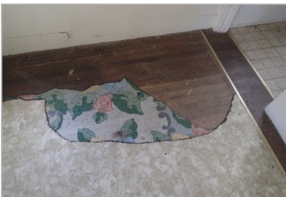
View of multiple layers of floor coverings that have crumbled away to expose the original wood floor below. Sagging and sloping of floors and evident wall cracking suggest the foundation has settled over time.
