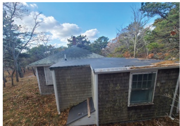
View of East elevation, there is a rear addition, with discoloration throughout siding indicating water damage.
