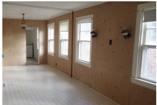
Floor to ceiling wood paneling with base and crown molting. There is some rippling indicating some deflection occurring from the interior structure.
