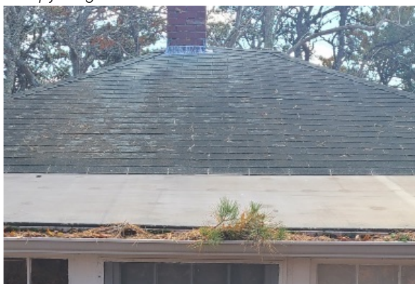
View of side addition membrane roof in relation to the original hip roof. The asphalt shingles are beyond their useful life. The gutter is filled with organic material supporting vegetative growth.
