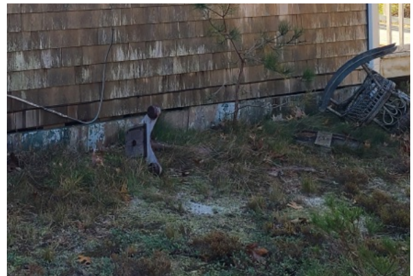
Rotting wooden foundation enclosure at grade.
