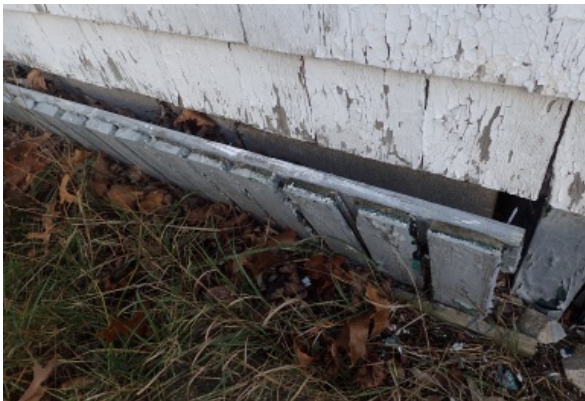
Wooden foundation enclosure rotting and detached from the building. Signs of past reinforcement efforts with a horizontal 1x3 can be seen at the very base.
