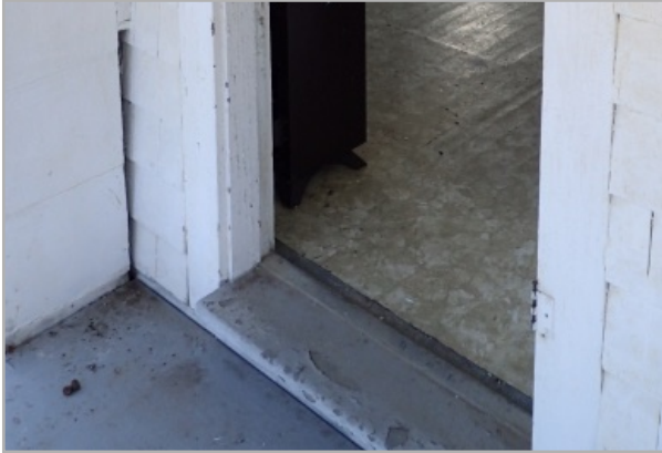
View of exterior threshold that is greater than one inch which is non-compliant with code, and deflection in the interior sheet floor finish can be observed.
