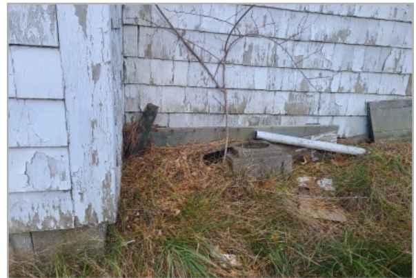
Ground and debris built up against CMU foundation and wall cladding at Southern elevation. Voids in the wall allow animals to enter and live under the building.
