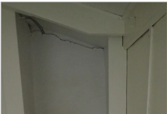
View of crumbling wall and ceiling due to insufficient moisture protection, and must be investigated for extent of damage.
