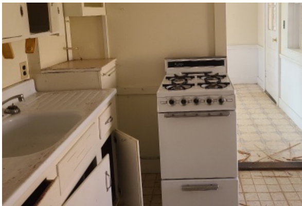
Stove/oven unit is outdated and needs replacing. There is no exhaust fan above the propane gas fueled burners.
