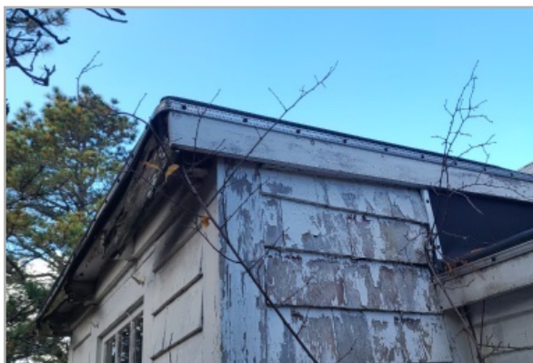
View of back additions, the membrane roof has failed and the fascia board has rotted out exposing the structure behind to the weather. The building siding has also been patched with a membrane sheet to the right.
