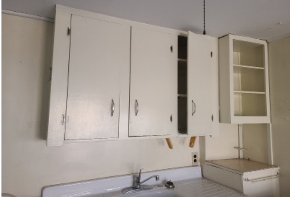
View of kitchen cabinetry and in counter sink. The hardware for the sink is non-compliant, and the cabinetry needs replacing due to structural concerns.
