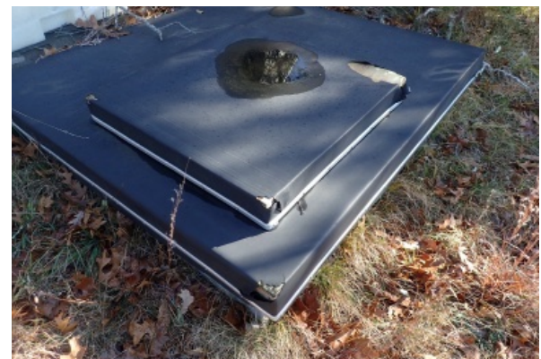
Membrane roof assembly nearby building similar to other membrane roof constructions on the property. Failure at the corners and edges indicates age and needs replacing.
