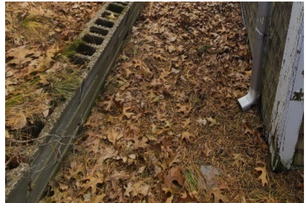
CMU retaining wall off set from foundation does not provide enough depth to keep the exterior building envelope from contacting the ground resulting in rotting and decaying of the exterior wall fabric in this location.
