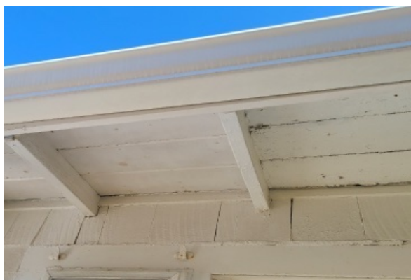
View of the roof eave condition where the paint is chipping between the sheathing boards. The peeling is not uniform throughout indicating that the roof eave may only have water penetration in just those areas.
