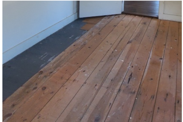
Buckled wood flooring in one of the bedrooms due to water damage.
