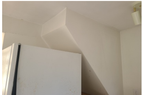
Sloped ceiling condition below stairs, enclosed with plaster and painted to match.
