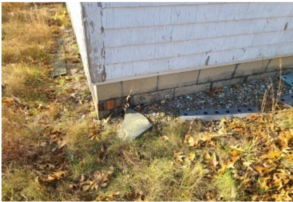
CMU foundation wall at grade, with brick patching seen in the corner.
