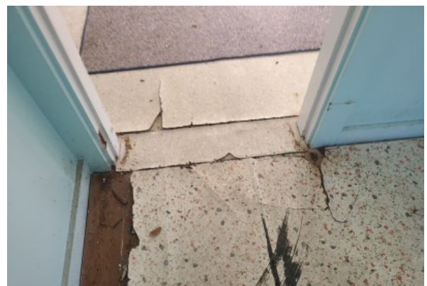
Piece made sheet flooring crumbling at the edges. Multiple layers of flooring can be observed in the area at the top of this photo. The area at the bottom has large areas where the flooring has crumbled to reveal the floor sheathing.
