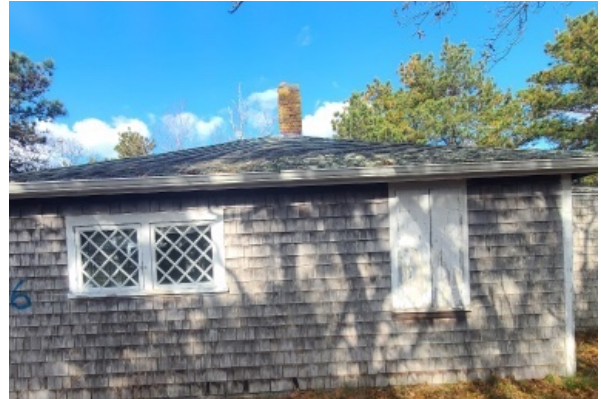
Southern face of the building, with one window opening boarded up. The sill of the covered window is rotted with signs that it is allowing water into the building.
