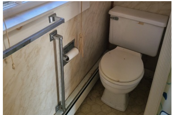
Toilet fixture with signs of damage due to normal wear and tear. There are nonconforming guardrails in this location as well.
