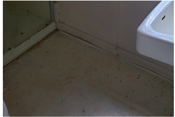
Sheet flooring in bathroom with signs of degradation throughout and crumbling at the edges. Signs of water damage are apparent at the edge of shower stall.
