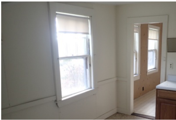
Painted plaster wall with trim about openings and at the base, as well as trim board at about 3' above finish floor. Paint shows signs of mold and mildew growth.
