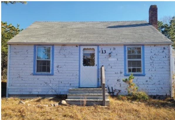
Front elevation of the building, concrete steps with insufficient railing, and original windows that need replacing.
