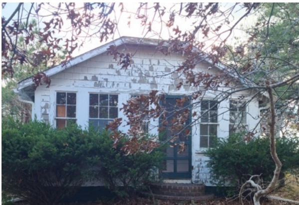
Front addition. Brick mortar steps, and peeling paint on shingle siding and fascia, rake, door and window trim boards.
