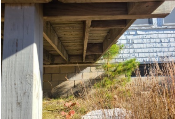
Deck addition framing supported by the CMU foundation at one side and piers at the other.
