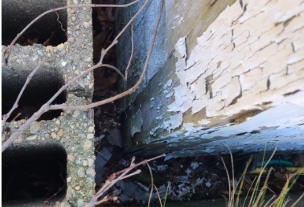
View of CMU retaining wall slightly offset from building siding. Paint has peeled from the base of wall up, indicating water has penetrated the CMU to the siding.
