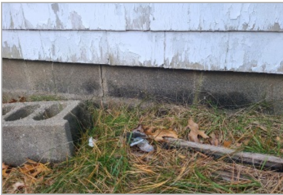
CMU foundation with discoloration indicating water damage within, and cracking in the mortar joints.
