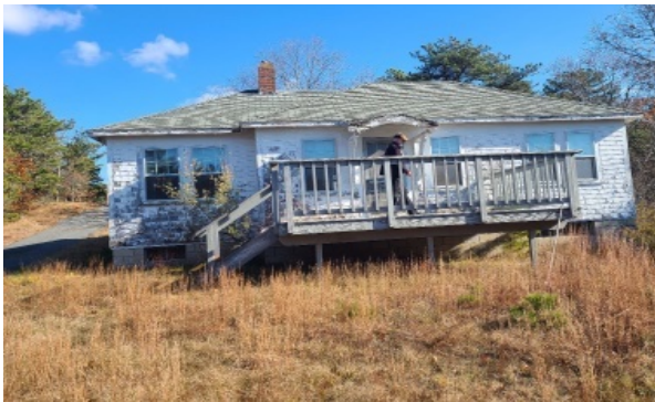
Shingled eyebrow canopy over front entry is rotted and failing. The fascia board is damaged and rotting at the entire perimeter of the roof. The wood deck is not worth saving.
