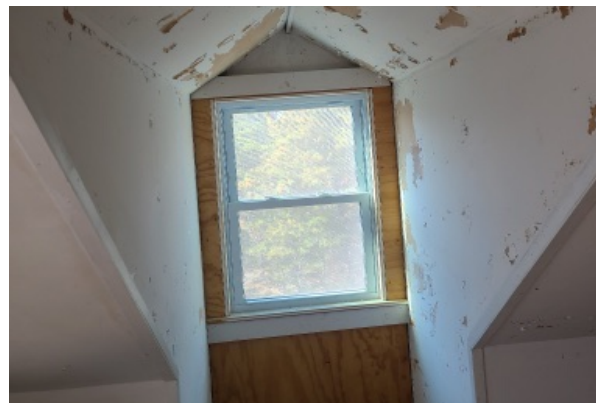
Dormer condition at the second floor. Chipping paint and insufficient framing about window.
