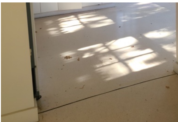
Uneven flooring transition between two rooms.
