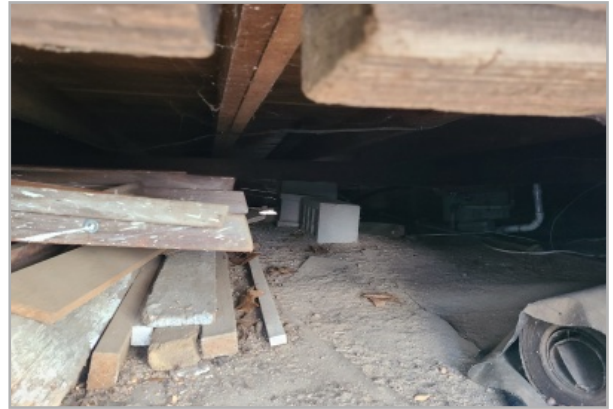
View to crawl space showing notched 2x6 beams and 2x6 wood floor joists. The exposed underside of this and many of the other cottages creates a potential habitat for wildlife.
