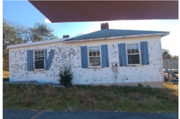
North elevation, bedroom addition to the left has with damaged window and peeling paint.
