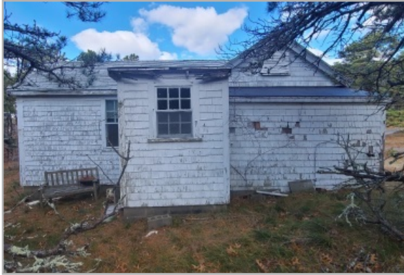
South face of the building, the paint is peeling and chipping on almost 80% of the wall surface area.
