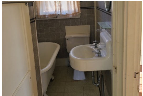
Full bath with toilet, sink, and bathtub. Sink fixture is non compliant, and bathroom layout is unacceptable by code.
