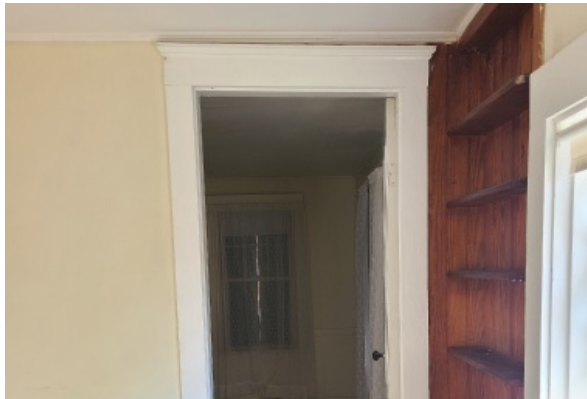
Interior door frame that is tilted, illustrating the failing foundation. This entire front room is sloping out from the central point of the inner most wall (facing here). The door opening width is 26\"/>
