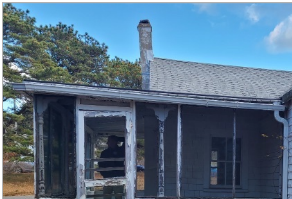
The front porch addition roof is pitched incorrectly causing water to run towards the gable end of the roof.. This entire construction has degraded and must be demolished.
