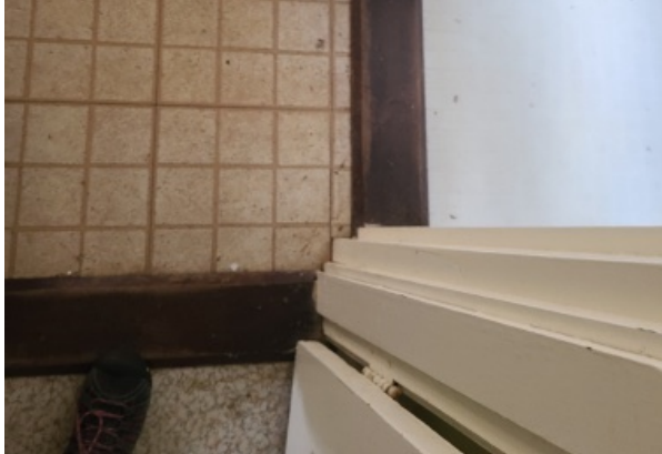
Condition of floor finish transition. Floor plan at this location is not wheelchair accessible due to configuration of cabinets and doorways and door thresholds.
