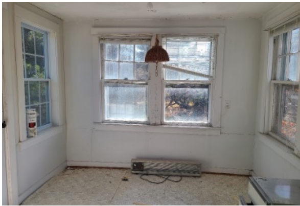
Kitchen addition, paint is chipping and peeling throughout and water damage can be seen at the windows.
