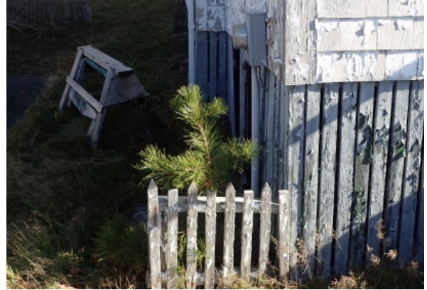
View of the foundation enclosure at the front of the building where the grade is the lowest. The boards of the enclosure are rotting and two layers of paint can be seen peeling.
