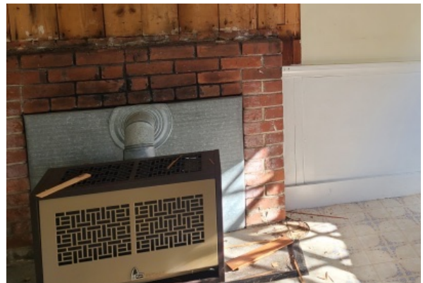
Propane fueled central heating unit with signs of water damage from the chimney.
