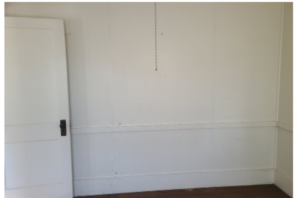
Painted plaster wall with corner and base trim, with trim board at about 3' above finish floor. Paint shows signs of mold growth and the seams between panels have become visually apparent.
