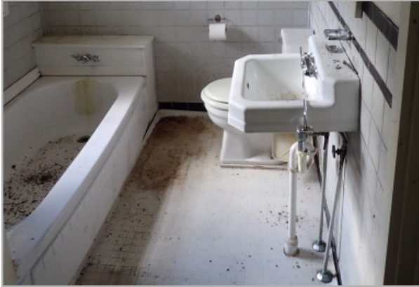
View of bathroom with non-compliant sink fixture, a bathtub with non-compliant hardware, and an outdated toilet that needs replacing.
