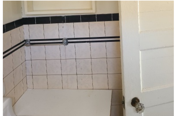
Tile wall finish in half bathroom, terminating in a tile bull nose and has painted plaster above.
