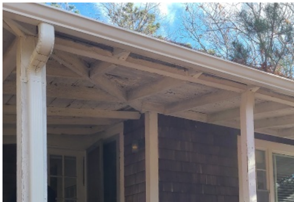
Front porch addition roof is an extension of the original roof and is secured into the exterior wall structure. The building structure is insufficient to support the porch canopy weight
