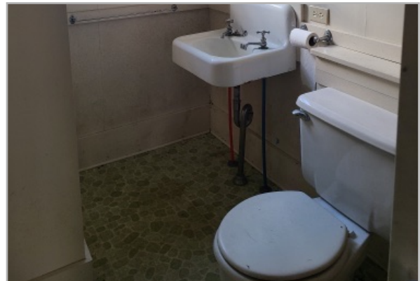
Wall hung sink with separate hot and cold faucet fixtures. Hazardous non-GFCI, non-grounded electrical outlet next to sink.
