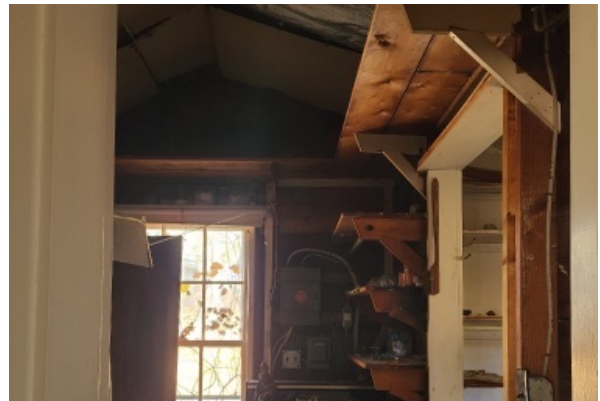
View into side addition, walls lack interior finishes revealing open stud bays without insulation.
