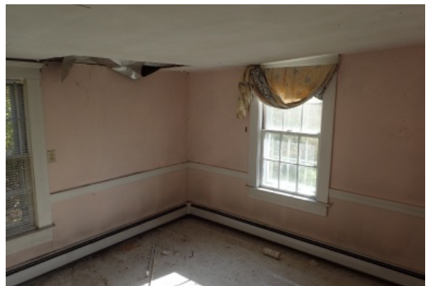
Painted plaster wall with trim about openings and at the base, as well as trim board at about 3' above finish floor. Paint shows signs of mold and mildew growth. The very low 6'-10" ceiling is open to the roof structure in one area.
