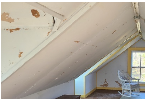
Roof from the interior of the second level. Water damage can be seen, as well as ripples indicating further damage and settling.
