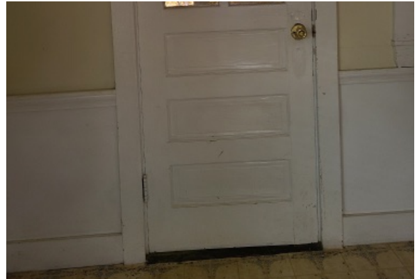
Door threshold in relation to the floor deflection, indicating a sloping settling foundation.
