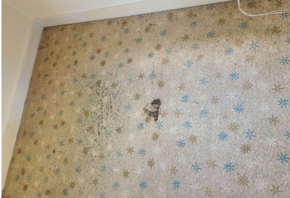
Sheet flooring, worn down to the floor sheathing in areas and crumbling at the edges.
