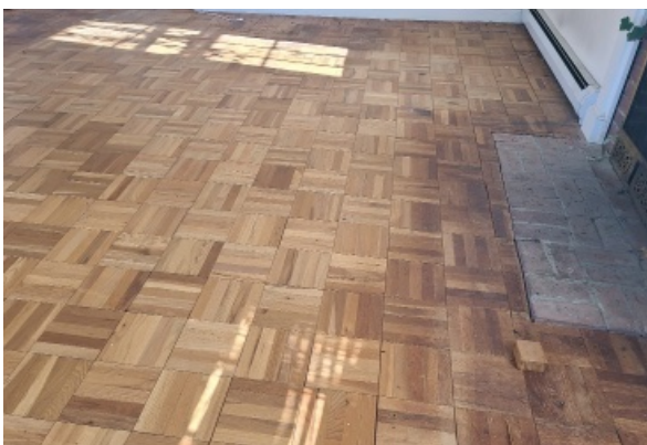
Wood parquet tile flooring with signs of warping and deflection throughout. Asbestos was dedected in the flooring.
