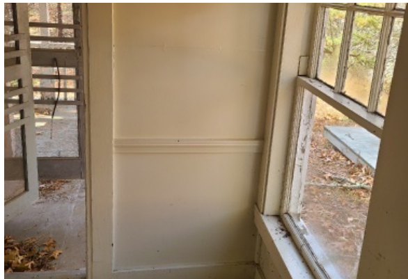
Exterior corner of side addition with painted plaster walls. The window is not protected with a storm window and is in poor condition as a result.
