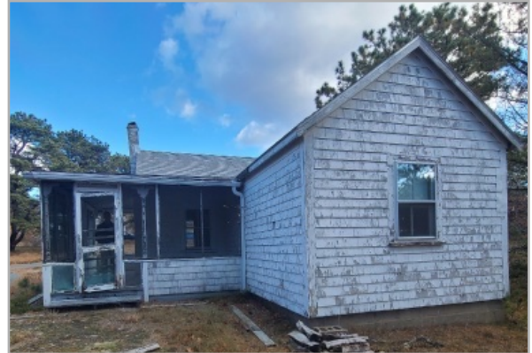
View of West face of building, the paint is peeling and chipping off of almost 90% of the surface area. The front porch addition is failing as is the masonry chimney.
