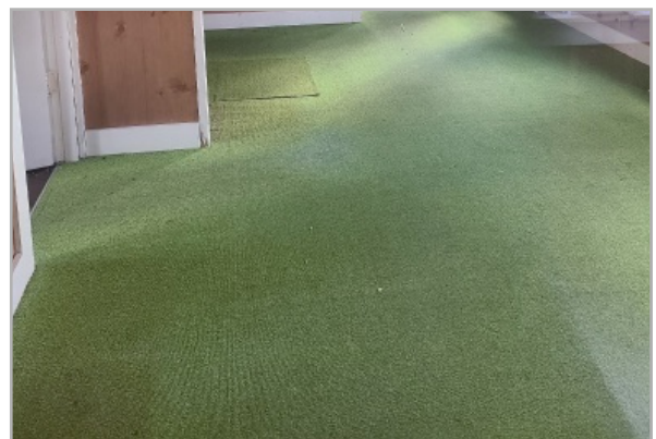
Synthetic grass carpeting covers a severely uneven wood floor surface due to sagging, undersized floor joists and foundation settlement. .
