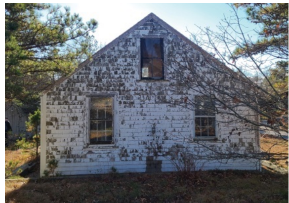
North elevation, cladding shows mold growth and paint has peeled from almost 50% of this face.
