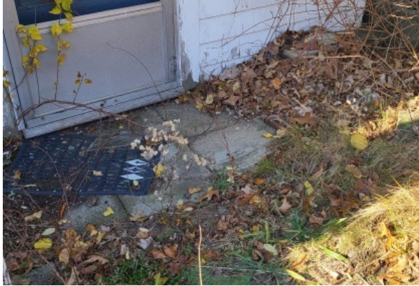
Concrete landscaping tiles at grade at the back entry to the building that have become obscured by the ground and vegetation encroachment and must be rehabilitated.
