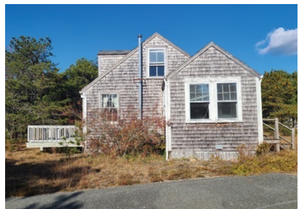
Unpainted cedar shingle siding in fair to poor conditons dependent upon wall orientation.
