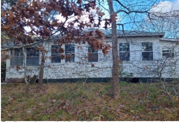
Peeling paint, and siding failing at penetration openings and rotting at the roof line. Additions to the left and right.
