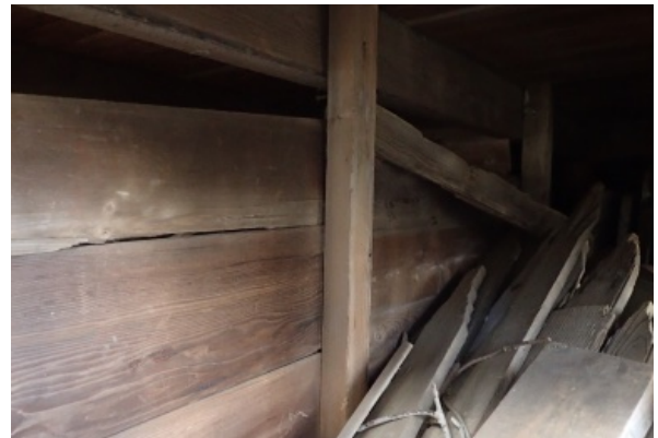
View into foundation crawl space. Insufficient floor supports can be seen, and a wood board partition dividing the space into storage and inaccessible.
