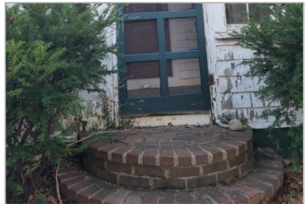
Brick steps at front entry. Note rotting shingles at bottom courses to brick.
