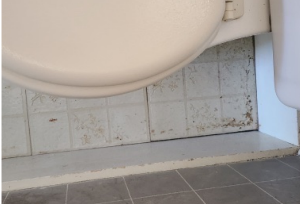
Sheet tile flooring in full bathroom. Tiles have become unsecured in areas and failing.
