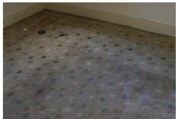
Sheet flooring in bedroom, evidence of water damage, and is crumbling at the edges due to age.
