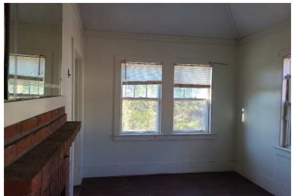
Painted plaster wall with base board trim and crown molding. Trim around window frame is beginning to separate from the wall, and needs replacing. Window hardware at the top is damaged and must be removed.
