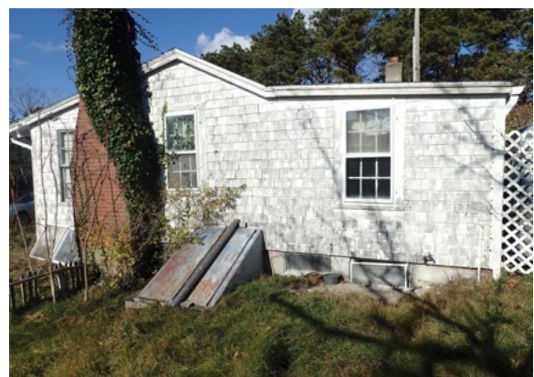
South elevation, vegetation penetration can be seen.
