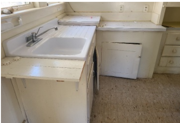
Counter sink, with non compliant hardware.
