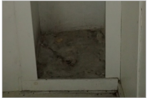
Bathroom flooring is sheet tile, and has areas of mold growth and discoloration. The floor of the shower stall and base of wall is covered with mold and mildew growth.
