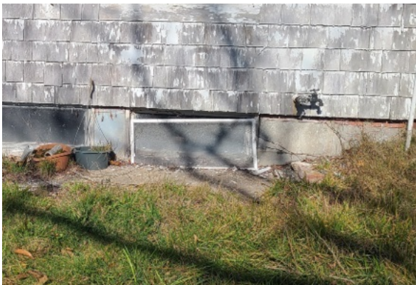
View of cracked parged CMU foundation. The basement window in this area is missing, allowing for animal habitation.
