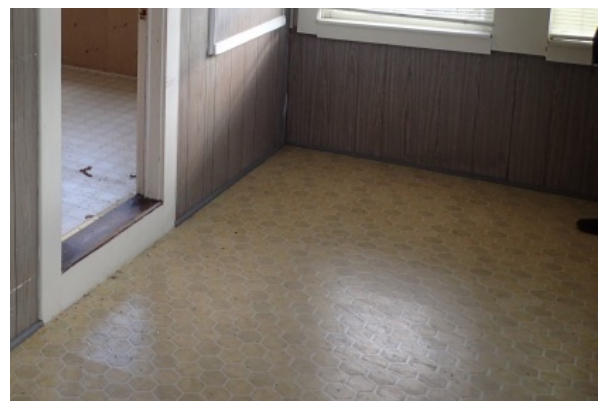
Change in material between rooms, and significant change in floor elevation. Floor sheet finish shows signs of deflections throughout.
