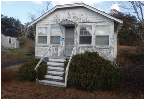
Front of cottage, front canopy roof assembly are rotted and insufficiently supported. Fascia board can be seen to be rotting as well.
