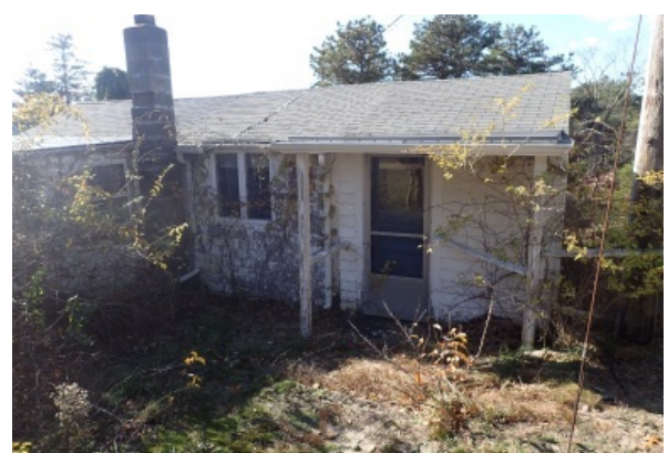
Rear elevation of the building where vegetation has penetrated the exterior chimney and into the building interior at open penetrations. Roof edge areas unprotected by a gutter lack paint and shows signs of decay.
