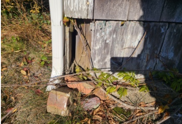
View of foundation pier, wood siding, wood foundation skirt, and brick supports. Foundation is insufficient for this building, and was not intended to support two levels.
