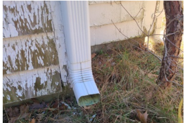
View of the base condition of a downspout where the last length of aluminum is missing. The water run off is insufficiently removed from the building footprint.
