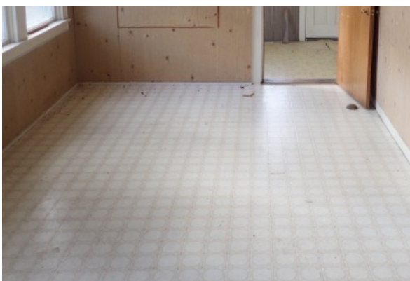
Wall to wall sheet flooring with word spots and some crumbling at the edges.
