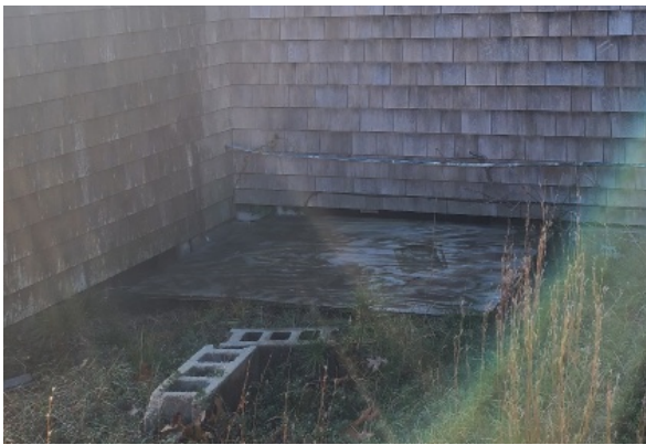
Rotting wooden access hatch to foundation crawl space, and remnants of CMU retaining wall.
