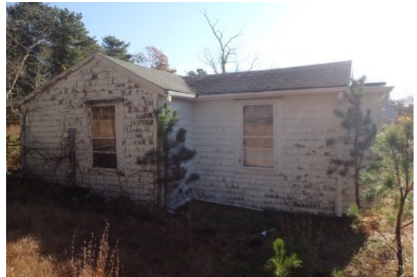
North face of building where exterior walls meets grade. Peeling and chipping of paint from the bottom up indicated water penetration from the base of wall.
