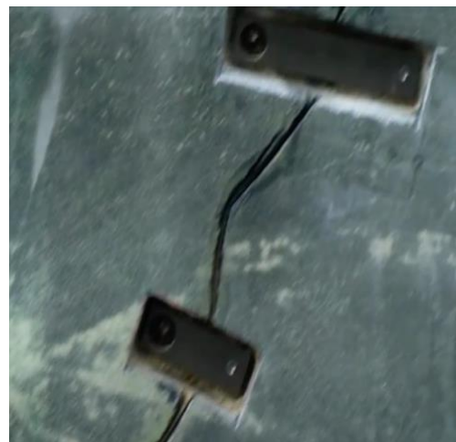
Images showing preparation and installation of epoxy clad, metal repair staples
