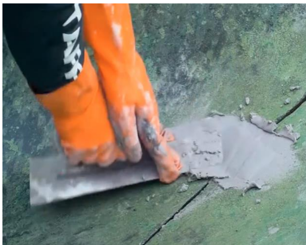
Images showing preparation and installation of epoxy clad, metal repair staples
