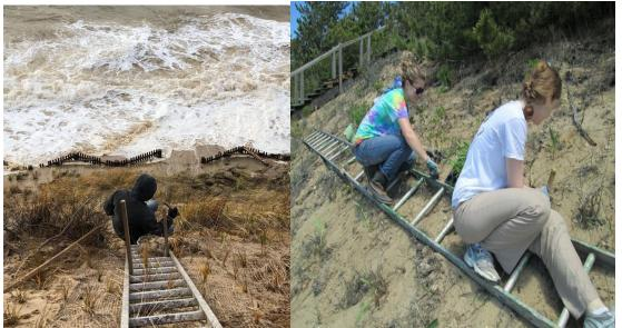
**6. Nourishment-** Bayside storm events can remove 1/3 cubic yard of sand per event. For any erosion control system applied to the coast, sand nourishment is required.
