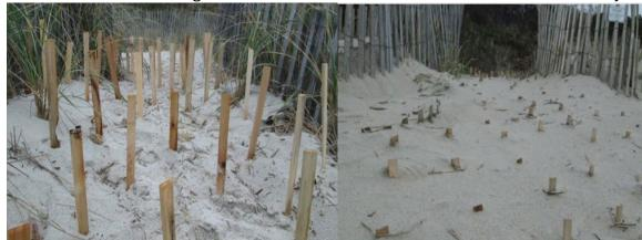
10. <u>Raised Walkways</u>- Access walkways in sand may require vertical clearance, for repositioning of sand elevations by wind. Excavation activity can generate impacts with spoil resettlement changing grade elevations and smothering native vegetation. <u>Recommendation</u>: we prefer using easy to install pin piles instead of excavation.
