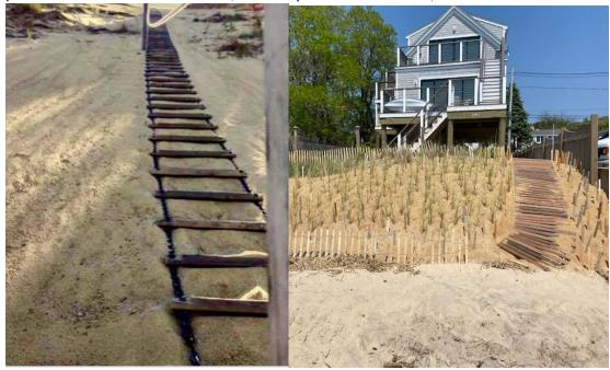
**12. Biomimicry-** Laminar surface flow winds are transporting sand from erosion areas. **Recommendation:** Storm winds that erode sand in one area, can deliver it to a deposition area, when exposed to turbulence inducing shims, which reduce velocity
