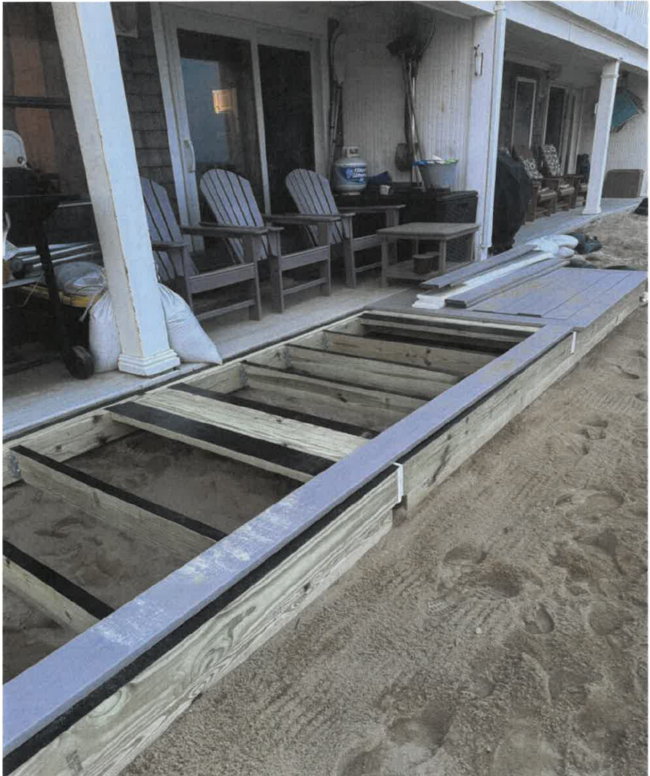
The deck consists of four sections approximately five feet wide by six feet six inches long—a total span of roughly twenty-six feet in length. This coincides with the length of the current deck to provide equal access.
