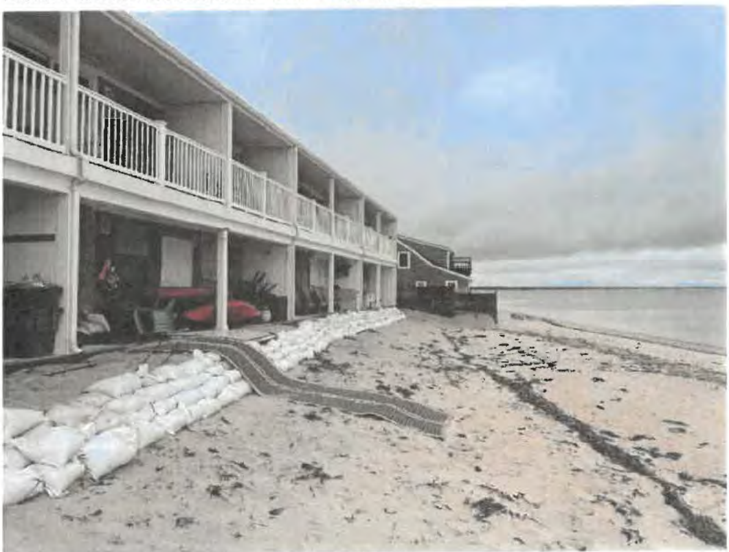
Photo 8: Coastal Dune conditions—east end (3/28/23)
