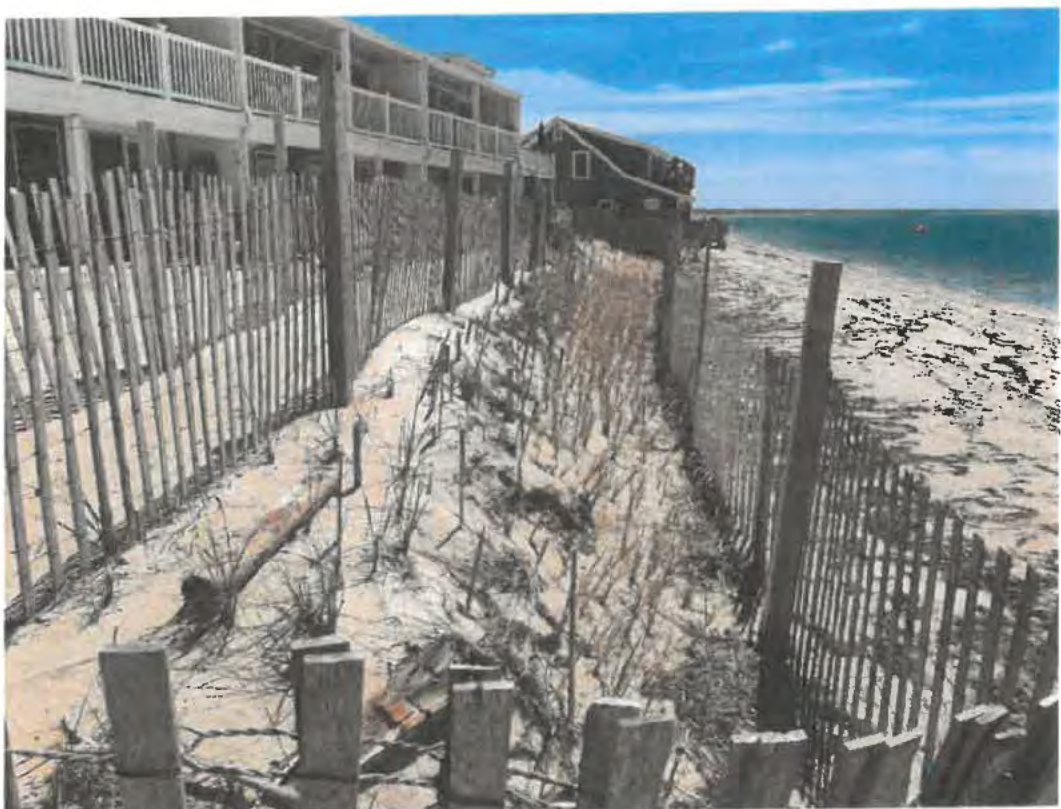
Photo 7: Coastal Dune conditions—east end (5/28/21)
