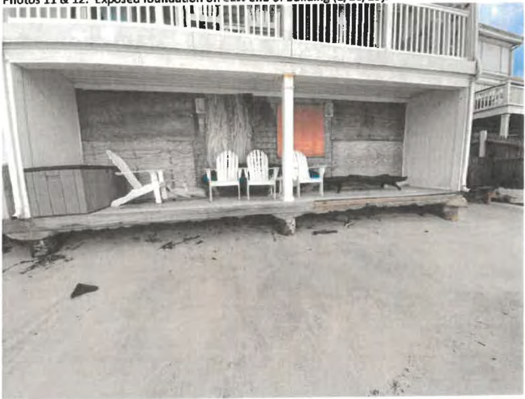
Photos 11 & 12: Exposed foundation on east end of building (1/26/23).
