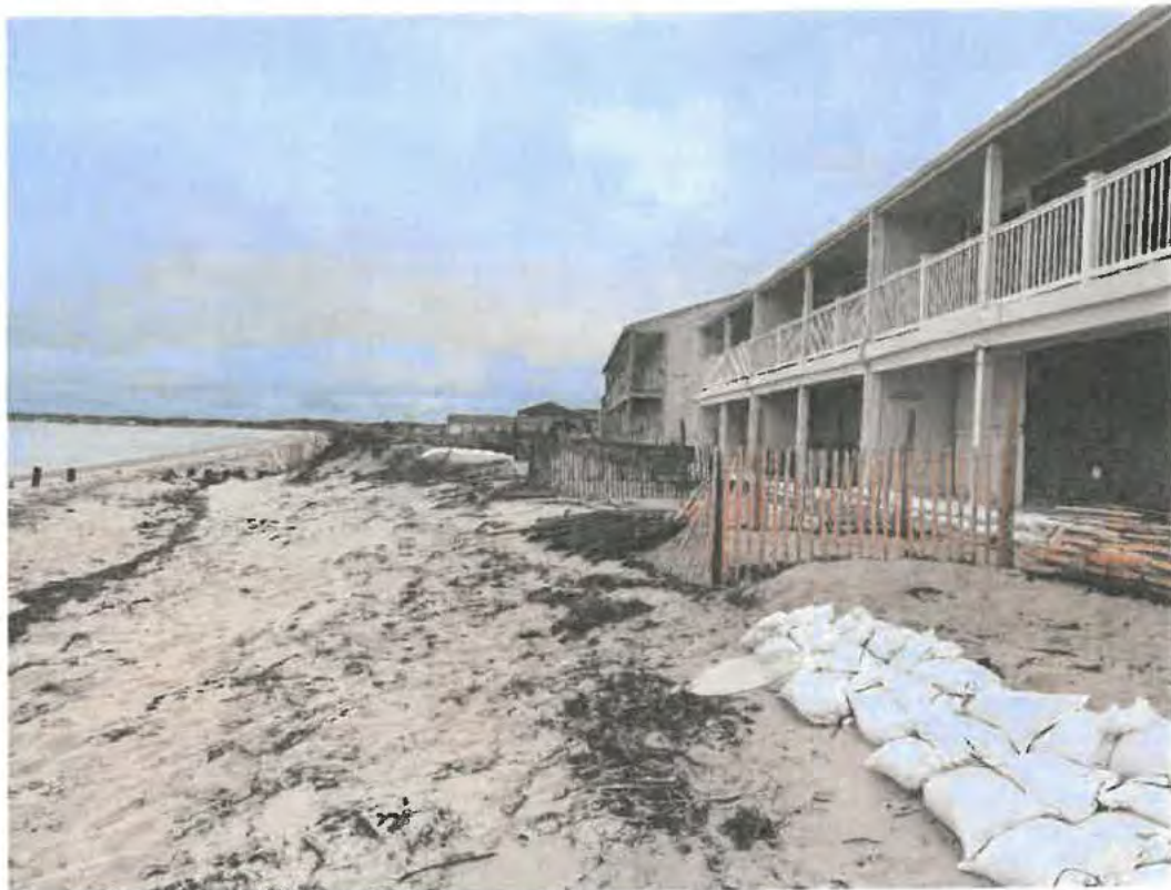
Photo 6: Coastal Dune conditions—east end (3/28/21)
