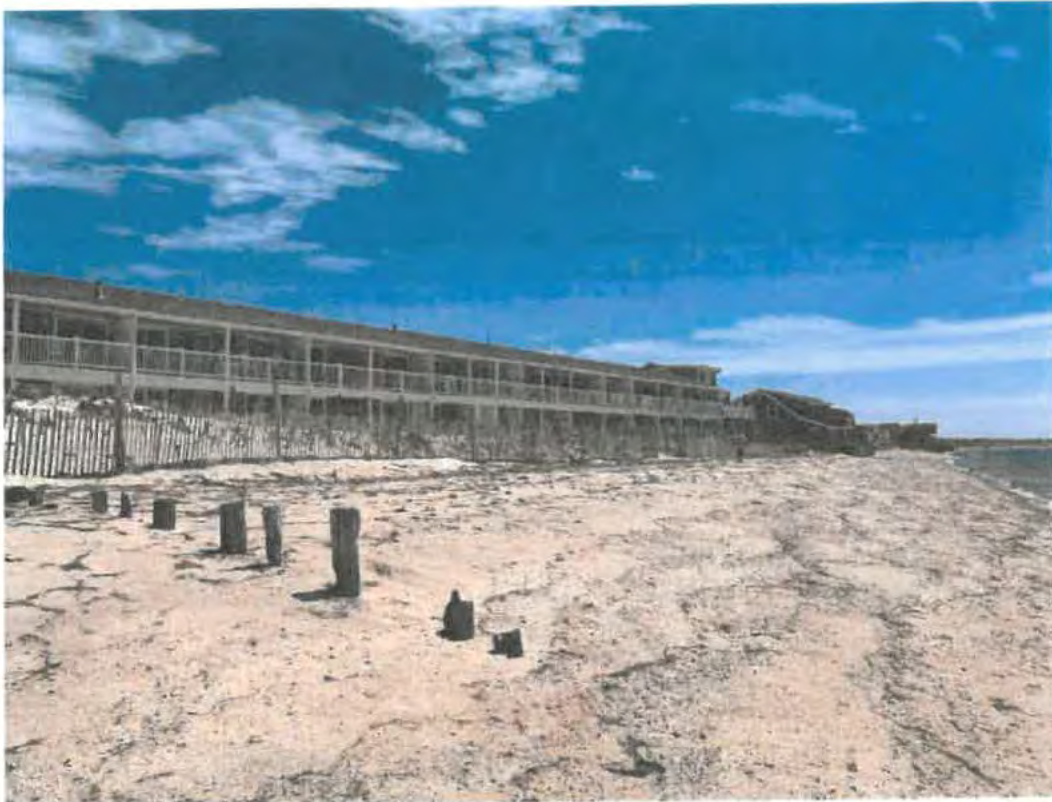
Photo 1: Northeasterly view of condos (May 28, 2021)
