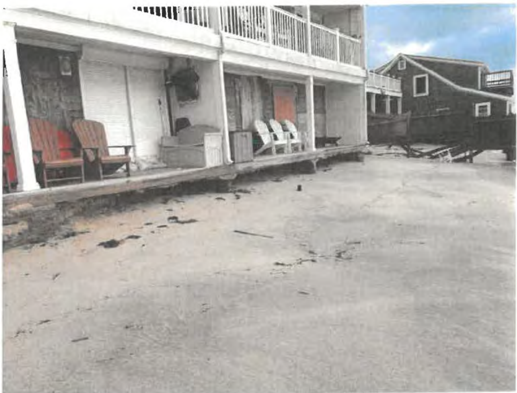
Photos 11 & 12: Exposed foundation on east end of building (1/26/23).
