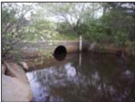
After crossing underground for approximately 375 feet the Pamet River emerges upstream of Route 6 through this 4-foot opening in the concrete headwall.
