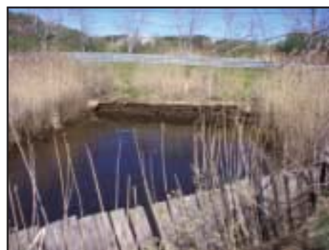
The 3-foot metal pipe and clapper gate set within this headwall (visible below the water line) pass only the seaward flow of the Pamet River under Wilder Dike (Truro Center Road/Route 6A).
