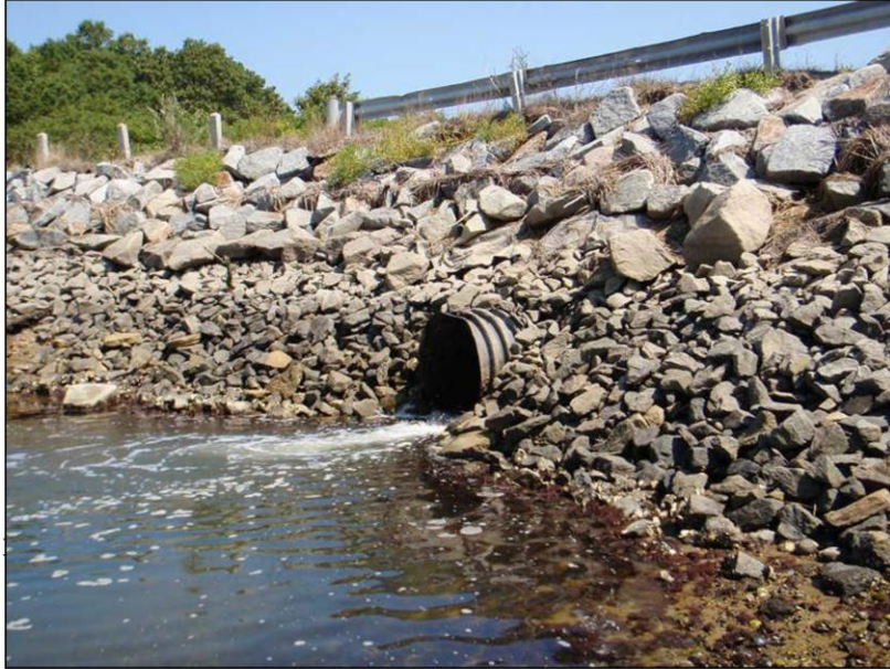
Figure MP1: Existing Culvert 3-foot culvert at Mill Pond and Mill Pond Road, Truro
