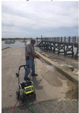
Water hose running length of gangway to dock for connection to ramp for power washing
